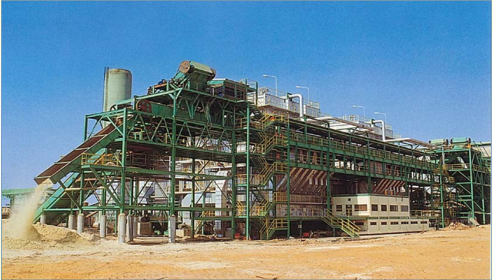
A bagasse firing boiler in a sugar factory of Thailand (300t/h 2units).
