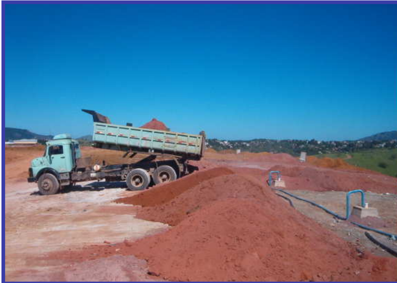
Landfill operator covering the site with soil
