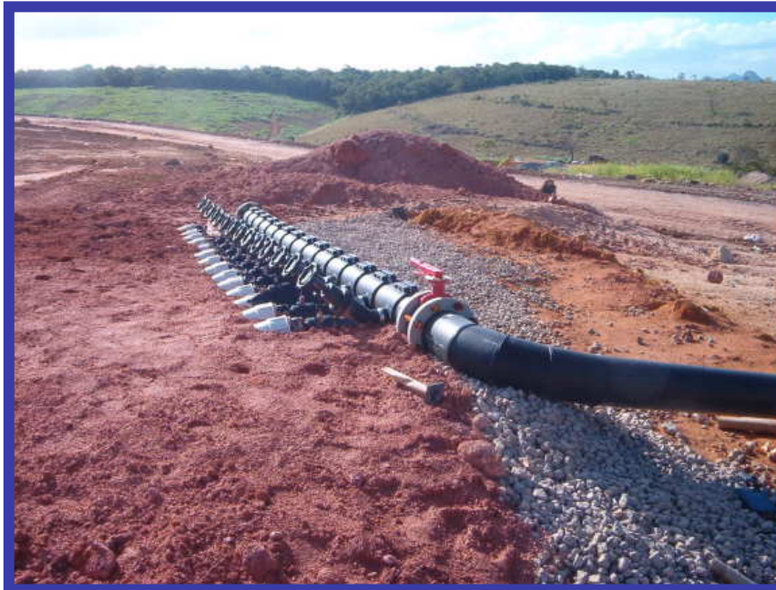
Manifold valves for balancing the landfill gas collection system
