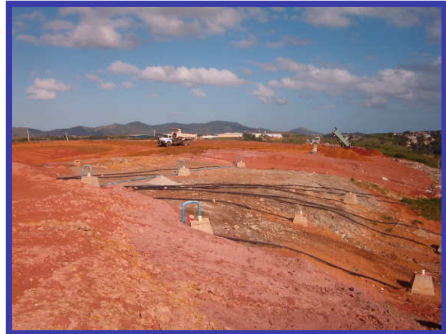
Installation of the landfill gas collection system
