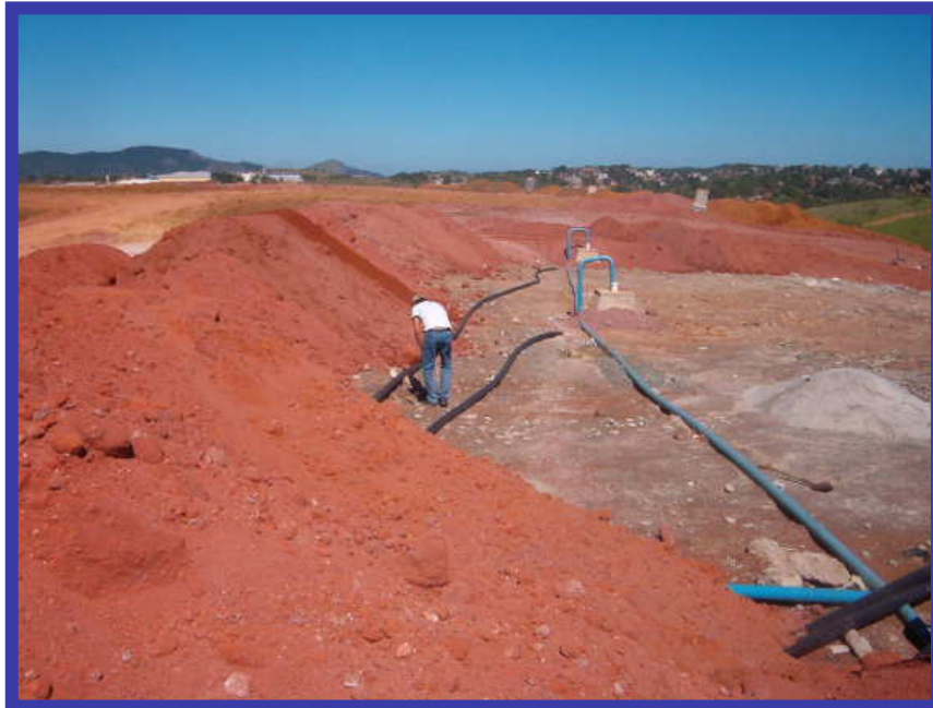
Installation of the landfill gas collection system
