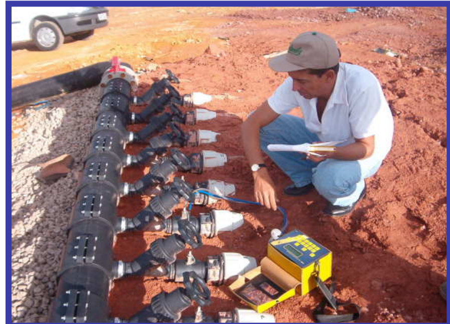
Manifold valves for balancing the landfill gas collection system
