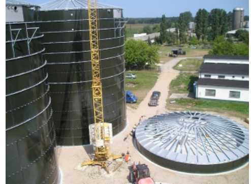
Photo. Biogas reactor before thermal insulation
