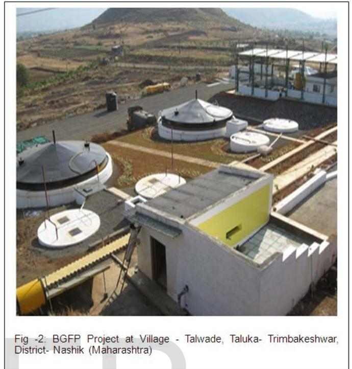
The biogas generated from the plant at vill.- Talwade, Dist. - Nasik (Maharashtra) by Ashoka Biogreen Pvt. Ltd. have been purified and a purity of 98.4% methane has been achieved through test conducted by Shriram Institute for Industrial Research, Delhi (NABL). The results are shown in Table 1.
