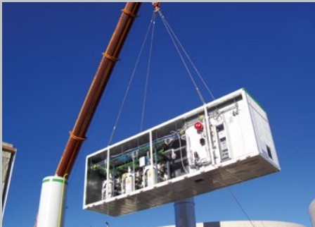
BGA 1000, biogas compression
