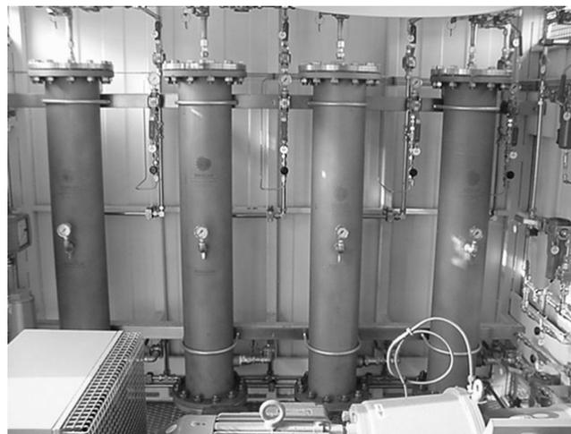
Figure 2. Four membrane units of the pilot plant
