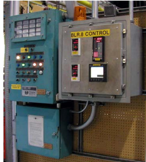
Simple BMS & Control Panel
