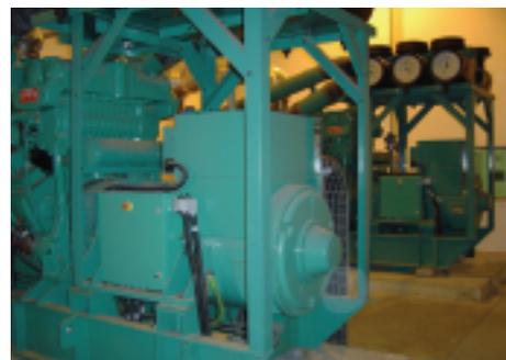
**The power plant consists of two 1370 kVA GQMA low-Btu generator sets, PowerCommand® controls, low-voltage switchgear and heat exchangers from Cummins Power Generation.**
