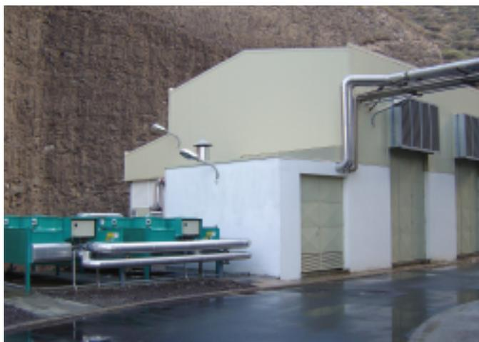
**The power building at Salto del Negro features a remote bank of radiators (left) to cool the generator set engines.**
